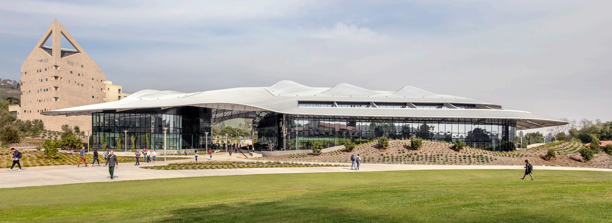
Cal Poly Pomona Student Services Building, LEED Platinum
