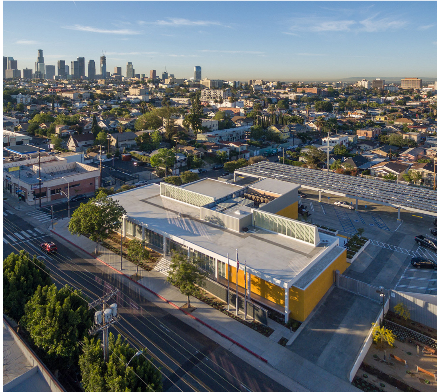
LAPD Old Rampart Police Station & Essential Facility Renovation, LEED Platinum
