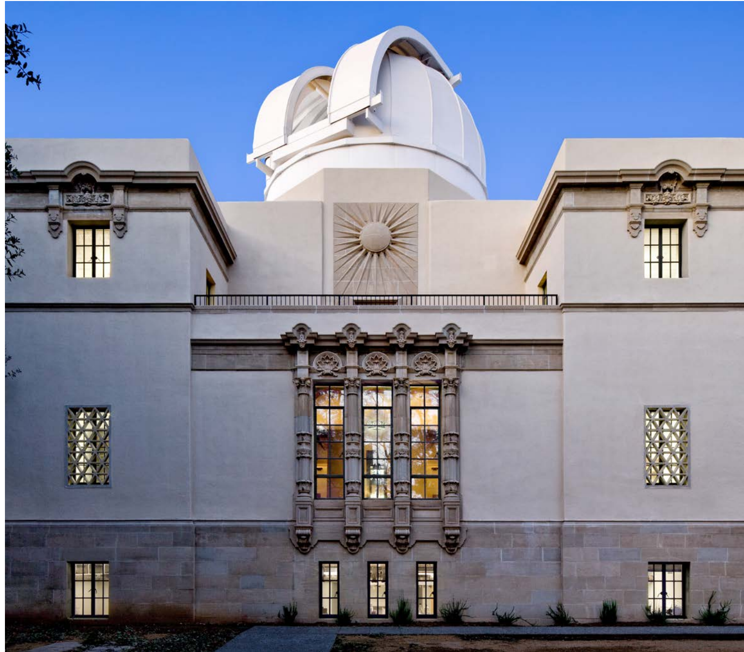
Caltech Linde+Robinson Laboratory for Global Environmental Science, LEED Platinum Nation's first LEED Platinum Laboratory in a Historic Building
