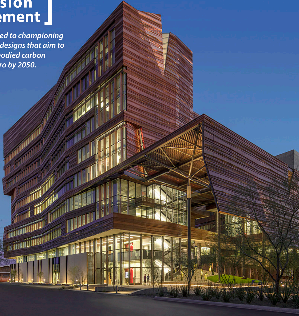
University of Arizona Bioscience Partnership Building (BPB) - Phoenix Biomedical Campus, LEED Silver
