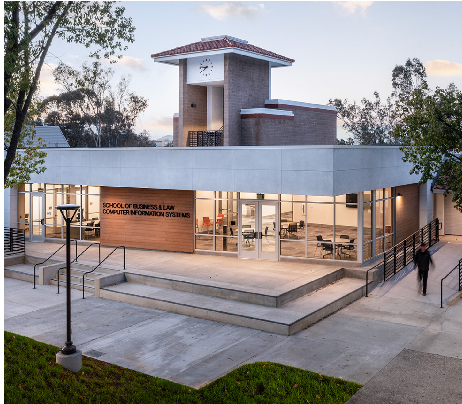
Riverside Community College District Reconstruction of Life & Physical Science Buildings, LEED Silver
